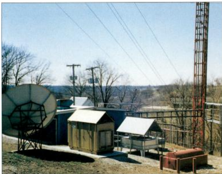
A typical transmitter site contains numerous potential hazards that, among others, may include falling objects, high voltage and fuel storage.
